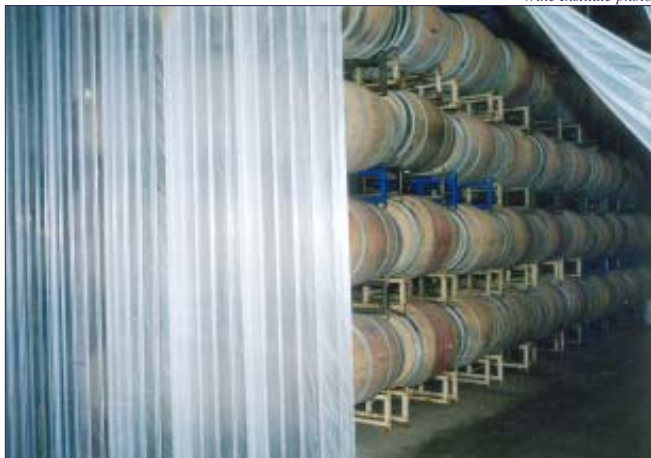
Plastic barriers help reduce energy costs by improving the efficiency of cooling systems in the barrel aging cellars at Buena Vista Winery in Sonoma.
