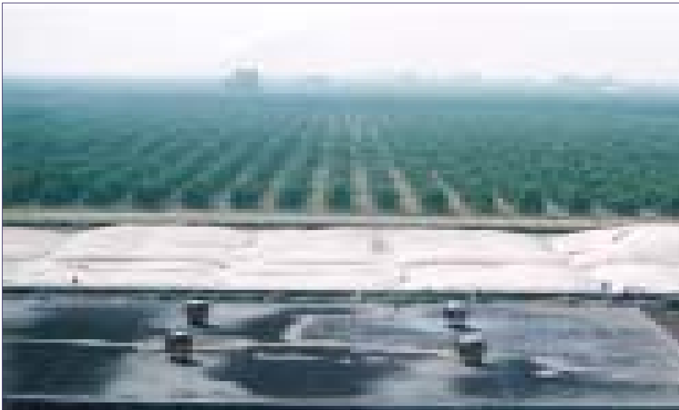
At left: A large membrane covering Sun-Maid's process water lagoon harvests the methane gas produced by the biodigester bacterium.
