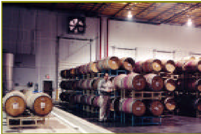
Temperature-controlled fans draw the cool air into Golden State's new barrel aging warehouse and distribution center in Napa, as General Manager Michel Blom checks on the energy-saving cooling system.
