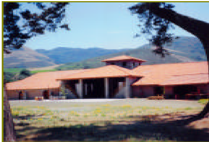
Above: Sanford Winery & Vineyards is constructed of thermal efficient adobe bricks to stay cooler in the summer and warmer in the winter.
