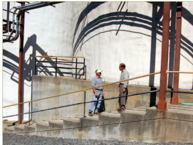
Korbel's investment in tank insulation had a two-year payback and helped keep the utility bill at the same level as five years ago, even with a 25 percent increase in production, says Bill Owens (right).
