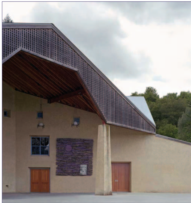
The thermal mass of Long Meadow's rammed-earth winery maintains a comfortable temperature year-round without heating or air conditioning. Long Meadow Ranch photo
