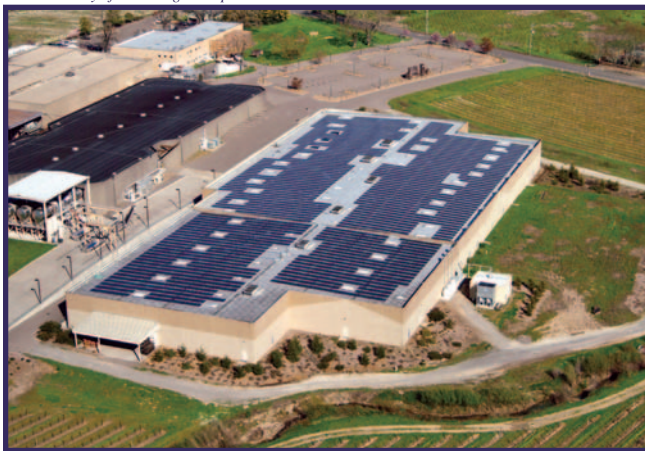
Fixed panels are mounted a few inches above the roof of Rodney Strong Vineyards' barrelhouse, ensuring that the system does not detract from the building's architecture while extending the life of the roof by shading it from UV rays and thermal exposure.
