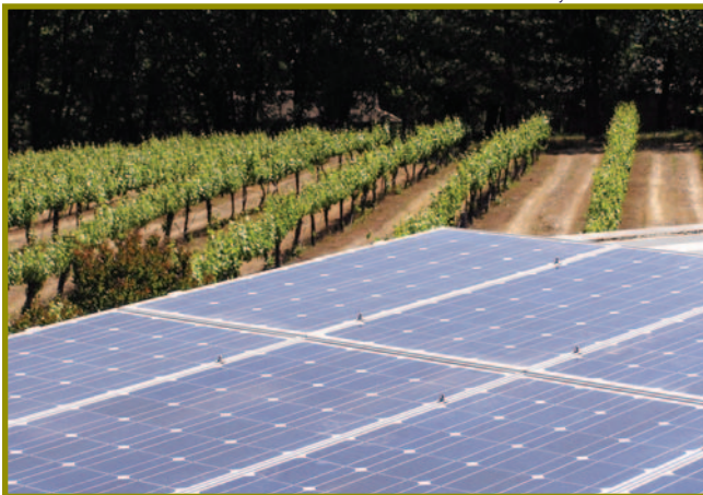
Like many California wineries, Sierra Vista Winery in Placerville decided to use solar energy because it matched the winery's goals for sustainable winegrowing.
