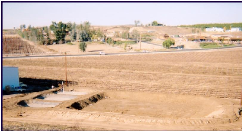
Shown under construction are Maurice Car'rie Winery's three settling ponds and a spreading basin for process water with wetlands habitat. The system is now nine months old.
